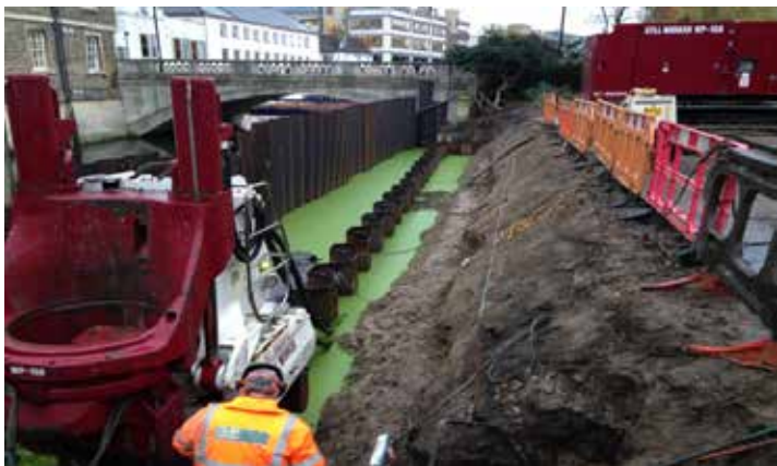
Traditional and Silent Sheet Pile Installation
