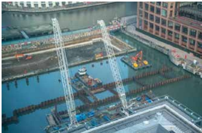
Piling and Cofferdam Construction
